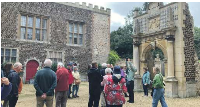
Courtyard, where part of the Elizabethan hall still stands
