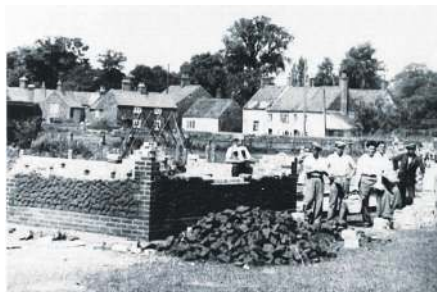
The Pavilion being built
