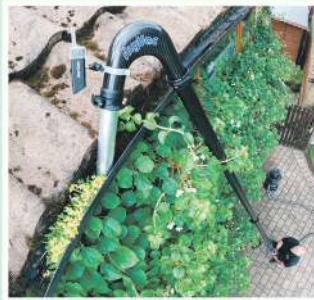
Gutter Clearing with SkyVac
