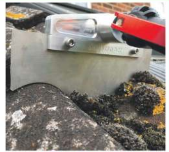
Moss Removal with Skyscraper
