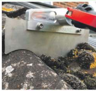
Moss Removal with Skyscraper
