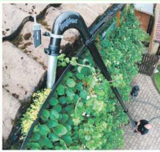
Gutter Cleaning with SkyVac
