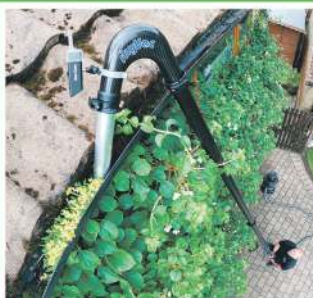
Gutter Cleaning with SkyVac
