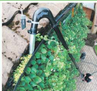
Gutter Cleaning with SkyVac
