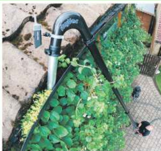
Gutter Cleaning with SkyVac
